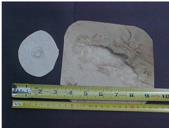
Photo 1: Small and large hail damage to two distinct PVC roof membranes
